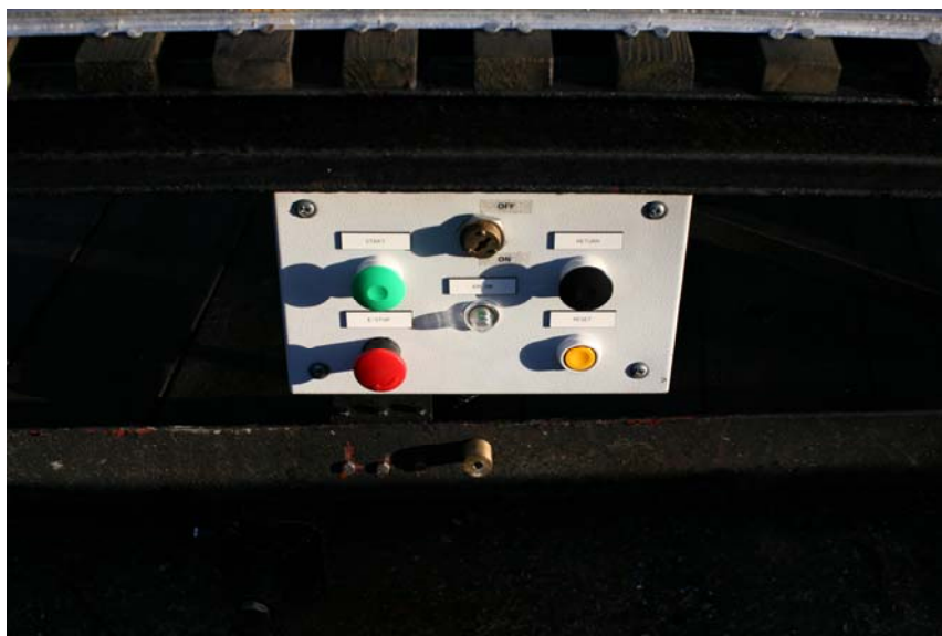
Picture Top: Season preparation sees George & Nick breaking the hard Russian coal Picture Middle: The recently completed pneumatic point as of last week Picture Bottom: A close up of the new control panel – a bit different to the old one
