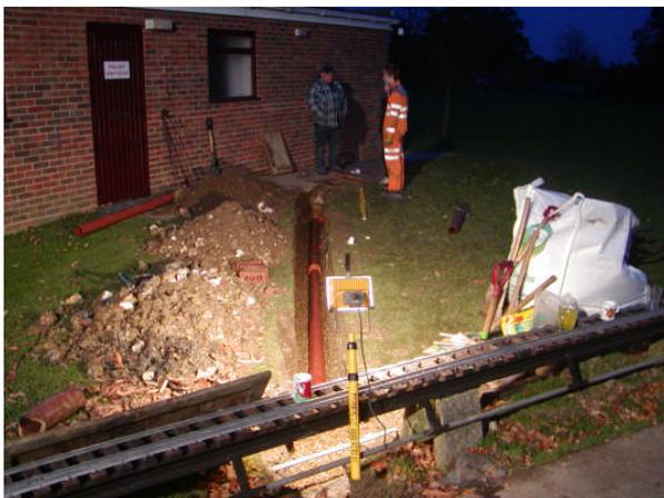
and laid plastic drainage pipe from the track to the man hole with a bend to bring it into the man hole and safely away. What should have been a fairly quick job, turned out to be about a months work! Still, it is done now and Ray has been busy mapping out the known waterways around the clubhouse and he will now draw up map showing these for the future generations!
