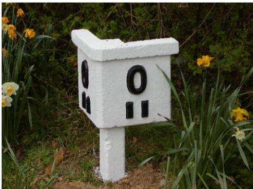
was actually in pretty neat order and just required a little touching in, here and there, to make it ready for painting. We used an exterior concrete paint which seems to go on quite well, you can get thick coverage and it is pretty quick drying, it will be interesting to see how long a water based paint lasts out in the elements though. The numbers were then painted in, in black gloss, trying to avoid any mixing with the white. With a
