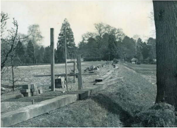
Laying out of Whittington Straight - 1952 (IPB-0275)
